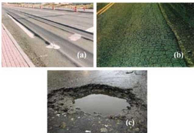
Figure 1: (a) Rutting, (b) Cracking and (c) Pothole deformations
