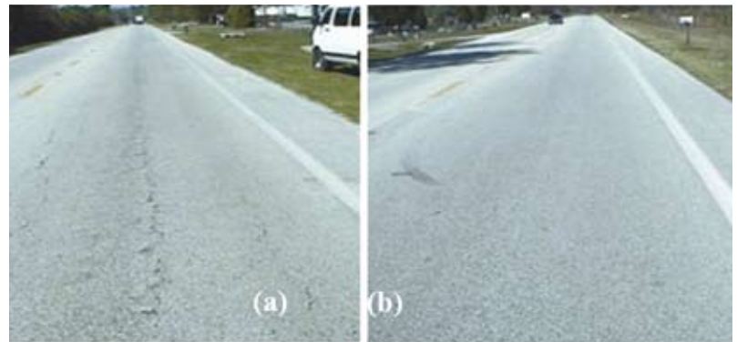
Figure 2: (a) Conventional Bitumen (Exhibits Cracking) and (b) Modified Bitumen (Without Cracking) [8]
